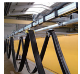
Flat cable and supports for cross travel
